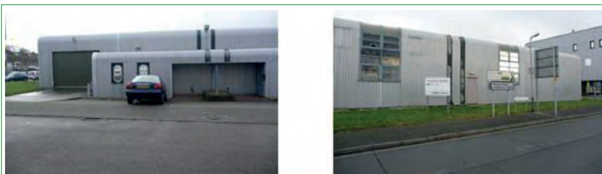
Fig. 108: Emplacement 30 – 36 Theaklen Drive, Zone Industrielle de Ponswood, Royaume-Uni (2013)
