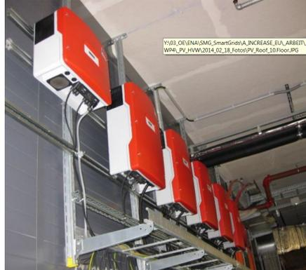
Figure 5.33: PV inverters, available at the 10<sup>th</sup> floor of the field trial building
